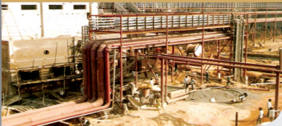
Rack Piping & Structural Works for Power Plant
