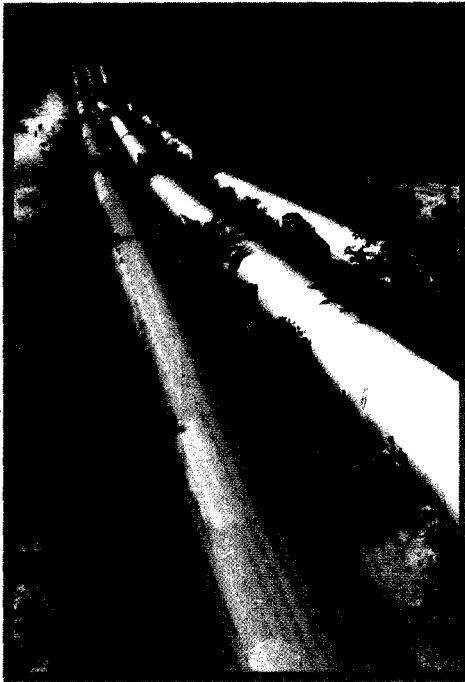
View of 1925 mm. dia M. S. Pipeline of T. K. Hally Project for Bangalore Water Supply & Sewerage Board.
