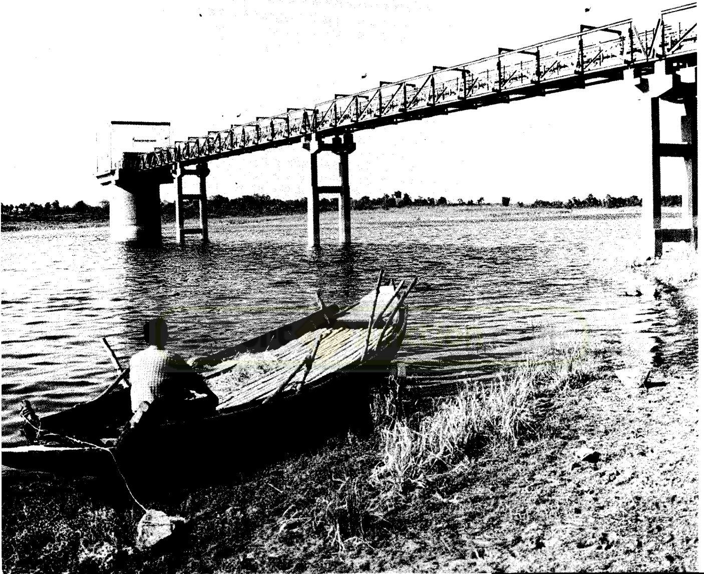
Intake Structure and Structural Bridge conveying Raw Water pipe over Utala River at Laksmampur for Raghunathpur Water Supply Project, West Bengal.
