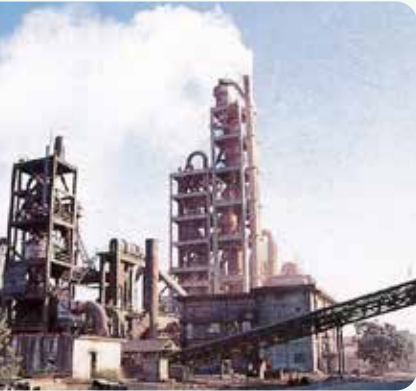
Installation of separate line calciner with five-stage pre-heater and jaw crusher
