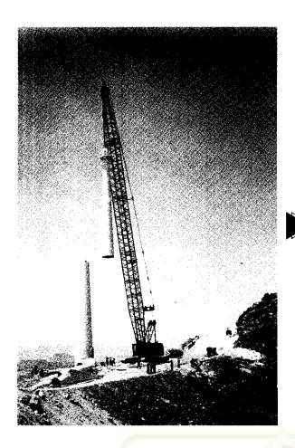
210 Ton Manitowoc 4100W Crane Series - 2 with Boom Length 210 Ft. carrying out Erection of Top Piece of E-40 Wind Fan weighing 28 Ton for Enercon (India) Limited at Chitradurga, Karnataka.
