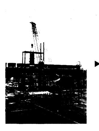
400 Ton Liebherr LG-1280 Crane with Main Boom 42 Mtrs. carrying out Erection of 80 Ton Waste Heat Boiler for Shut Down Job at Gujarat Narmada Fertilizers Company Limited, Bharuch, Gujarat.
