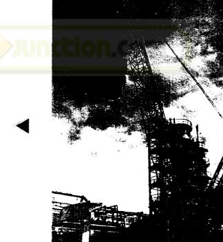
270 Ton Kobelco P & H 5300 Crane with Main Boom 60 Mtrs. carrying out Dismantling of old Vacuum Column weighing 140 Ton at Coker Revamp Project, Indian Oil Corporation Limited, Barauni, Bihar.
