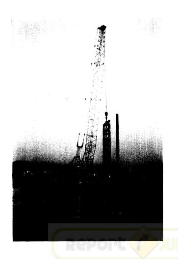
204 MT. American AH9310 Crawler Crane with Lattice Boom assembled with 160 Ft. Boom length to carry out Pile Driving Operation using Diesel Hammer for Skanska Cementation India Limited at Sea Bird Project, Karwar, Karnataka.
