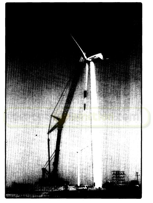
800 MT. Liebherr Telescopic Boom Crane erecting 1.25 MW. Wind Energy Generator of 74.5 Mtrs. Hub height of Suzlon Developers Private Limited at Coimbatore, Tamil Nadu.
