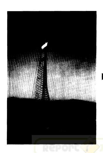
400 MT. Demag Crawler Lattice Boom Crane assembled with 90 Mtrs. Main Boom erecting 1.25 MW. Wind Energy Generator of 74.5 Mtrs. Hub height of Suzlon Developers Private Limited at Chitradurga, Karnataka.
