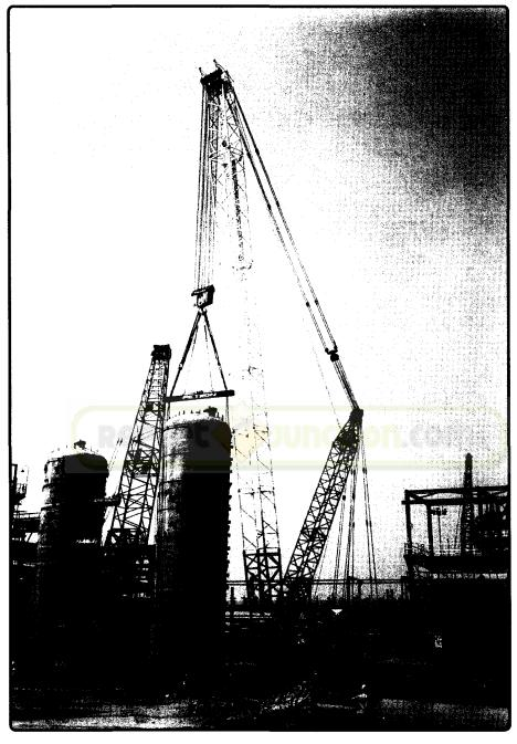
600 MT. Demag Crawler Crane in SSL Configuration with 90 Mtrs. Main Boom erecting 225 MT. Equipment Weight at Indian Oil Corporation Limited, Panipat Refinery, Haryana.
