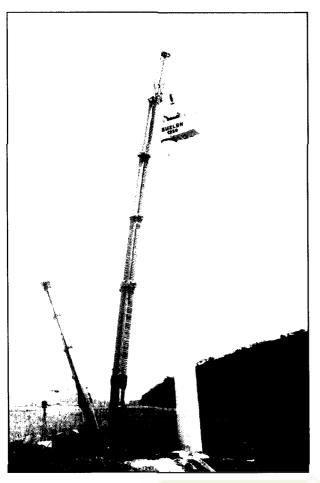
500 MT. Gottwald Truck Mounted Telescopic Boom Crane with 57 Mtrs. Main Boom & 10 Mtrs. Fix Jib erecting 1.25 MW Wind Energy Generator at Sogi, Karnataka.
