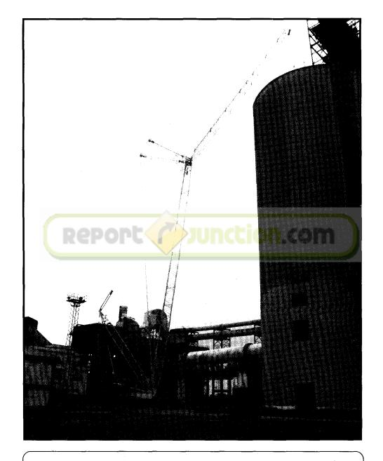
BRAND NEW Terex-Demag CC 2800-1 Capacity 600/800 MT Crawler Crane, assembled in 'SWSL' Configuration with 84.0 mtrs. Main Boom + 84.0 mtrs. Luffing Jib, carrying out the erection of string structures at Sanghipuram, Gujarat for Sanghi Industries Ltd. (We have 4 nos. such CC 2800-1 Cranes)
