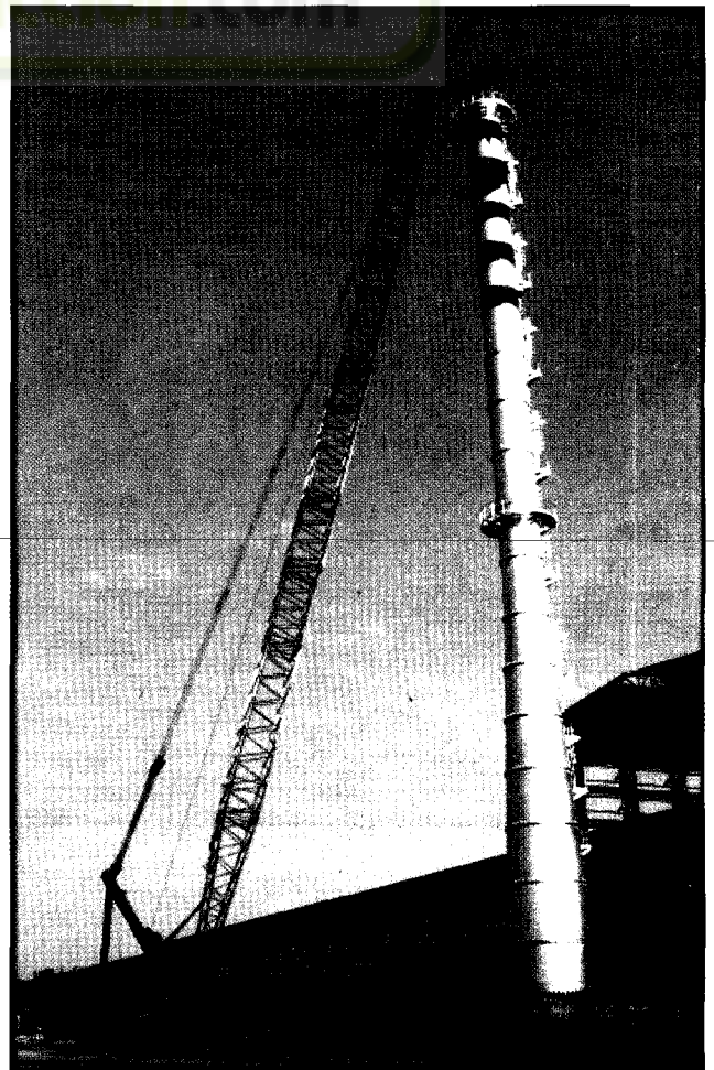
MANITOWOC M4600 S-3 , Capacity 275 MT, Crawler Crane assembled in with Main boom - 79.2 mtrs. & Fix Jib - 15.24 mtrs. Working for the STACK of 82 mtrs. Height for WELSPUN GUJARAT STAHRROHREN Ltd., Anjar, Gujarat.
