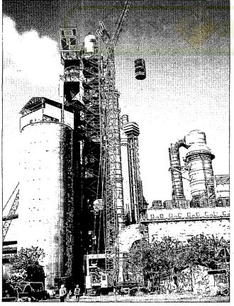
450MT DEMAG CC2400 Crawler Crane assembled in `LW' Luffing configuration with Main Boom - 78m + Luffing Jib - 72m (Total=150m), carrying out the erection of Cyclones & Structures of Pre-Heater Building at a Height 112m for LAFARGE CEMENT at Raipur, Sonadi, Chattisgarh.
