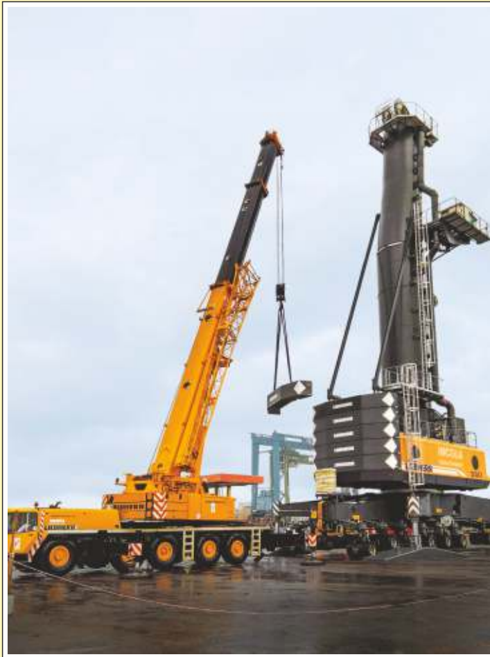
LIEBHERR LTM 1160/2 (Capacity : 160 Ton) All Terrain Tyre mounted Telescopic Boom Crane doing the erection & assembly of Liebherr Harbor Mobile (LHM 550 -141546) Crane for Tuticorin Port Trust, Tuticorin at Tamilnadu
