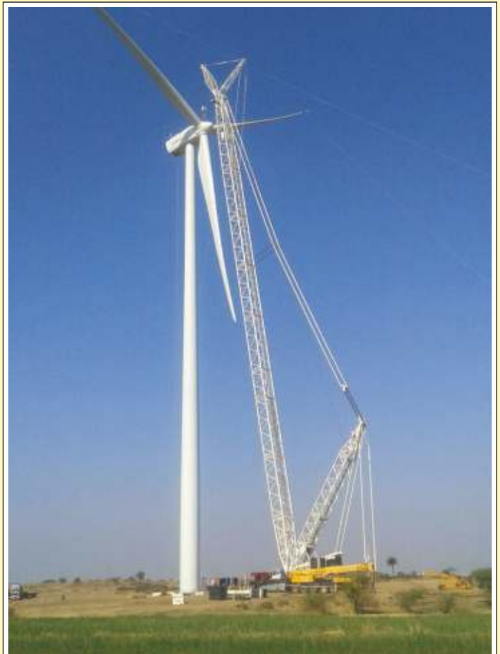
Terex Demag CC 2800/1 Crawler Lattice Boom Crane erecting 2 MW Wind Turbine at a height of more than 100 meters in Central part of India
