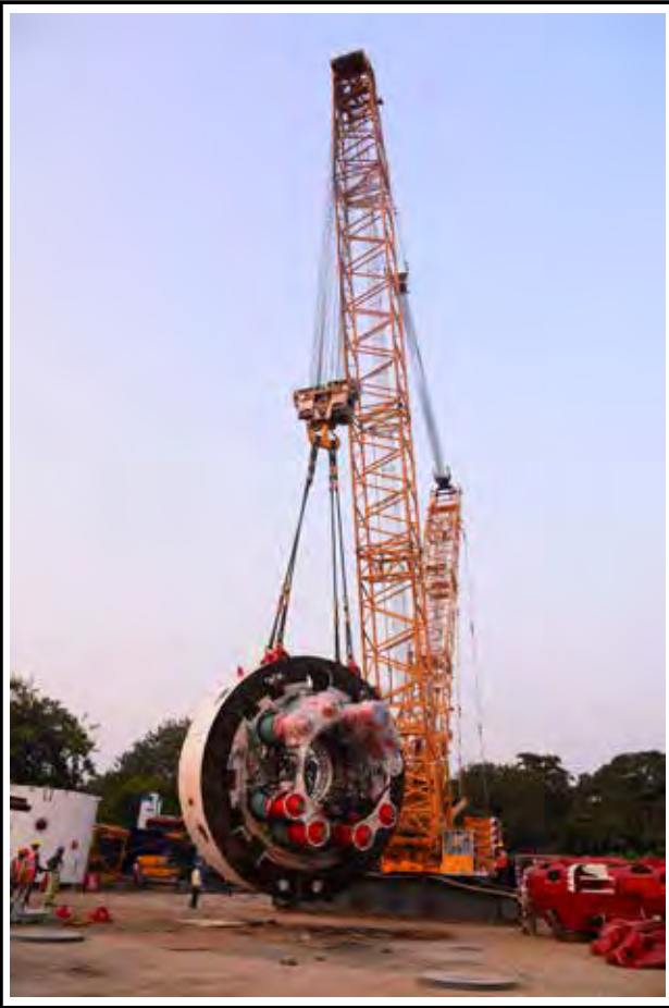
Liebherr LR 1400/2 SDB 35 m handling TBM components with a maximum load of 180 MT at MMRC, Mumbai.
