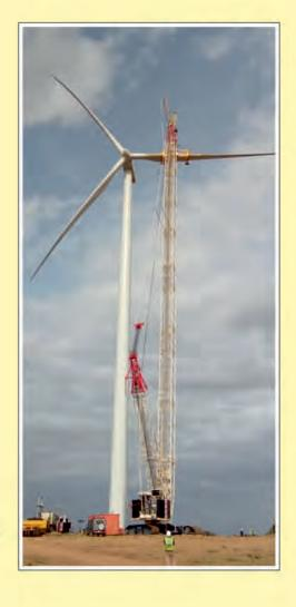
Blade Erection weighing 29 MT at 54 m using a 600 MT CC in Southern India.
