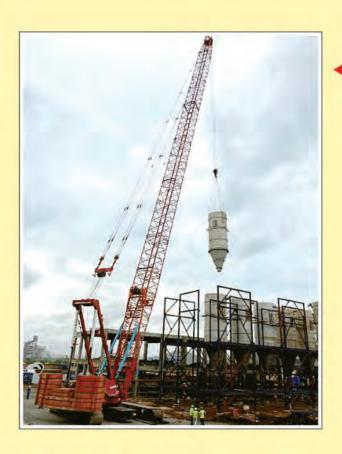
275 MT crawler crane deployed for erection work in a chemical plant in Karnataka.
