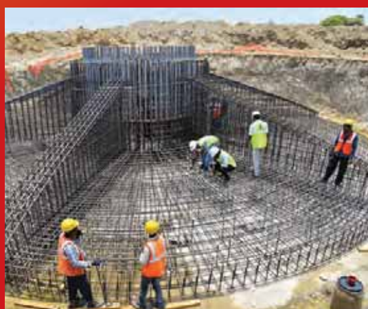
Wind Turbine Generator (WTG) Final Foundation at Sandur Karnataka
