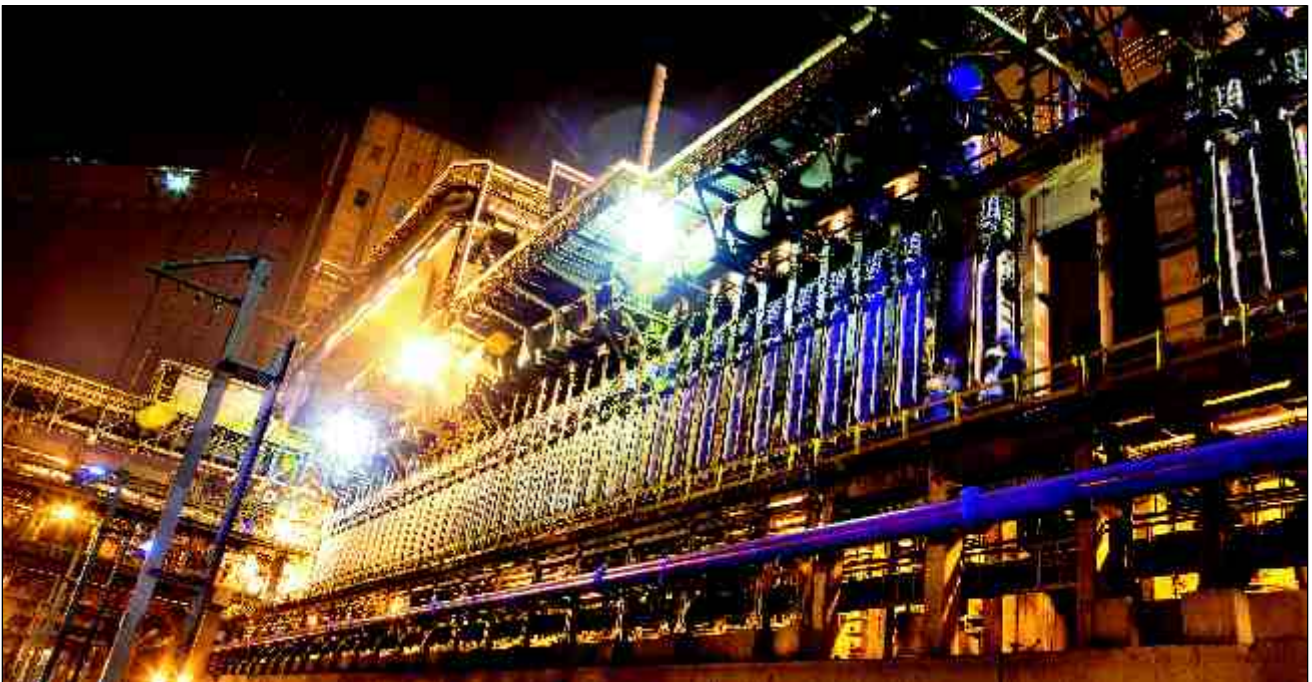
Coke Ovens Battery no. 2 at Durgapur Steel Plant
