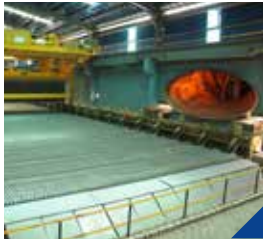
Cell house at Dariba zinc smelter, HZL
