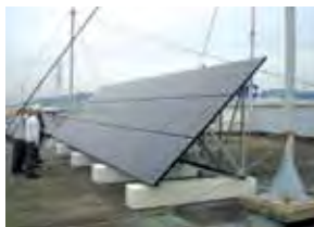
4kW Standalone Solar installation, Japan
