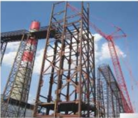
A view of transfer point erection in a CHP
