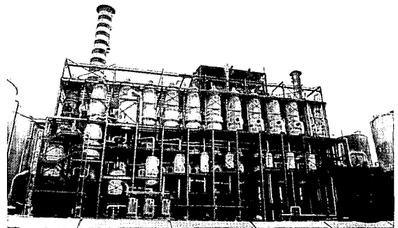
Multiple effect evaporator
