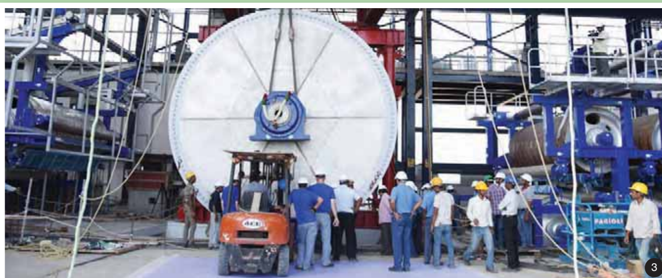
New Board Machine being installed in Mondipatti Village, Manaparai Taluk, Trichy District: (1) Wire Section (2) Dryer Section (3) MG Cylinder
