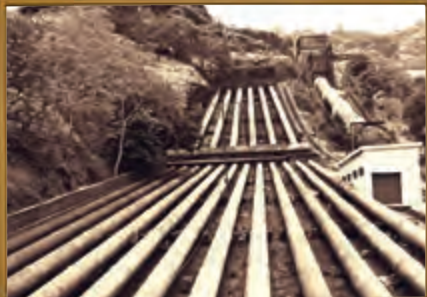
Pipelines to carry water to Power House
