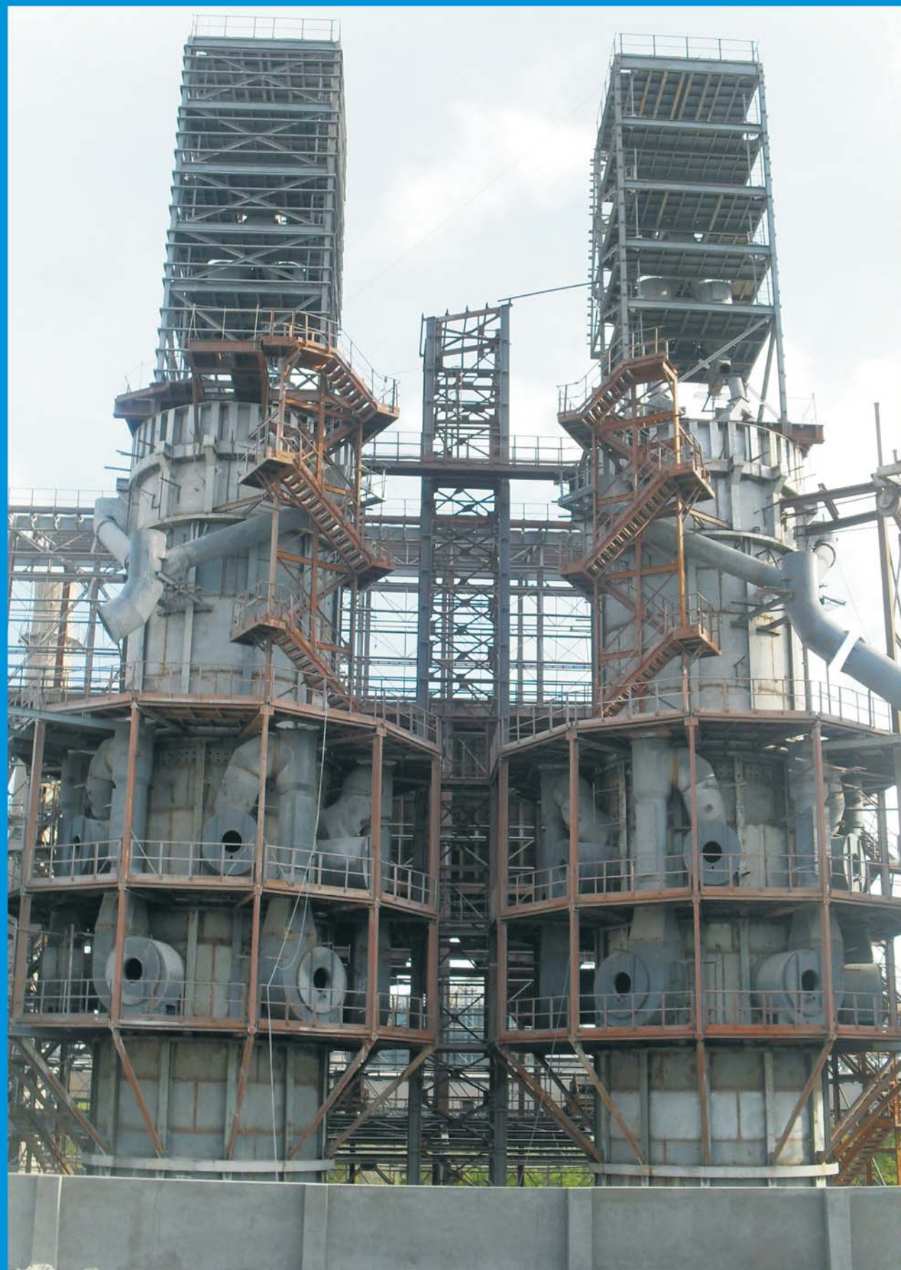
2 x 500 TPD Vertical Shaft Kiln under construction
