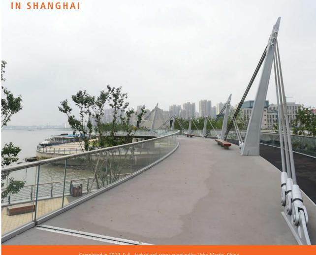
Completed in 2017. Full - locked coil ropes supplied by Usha Martin, China
