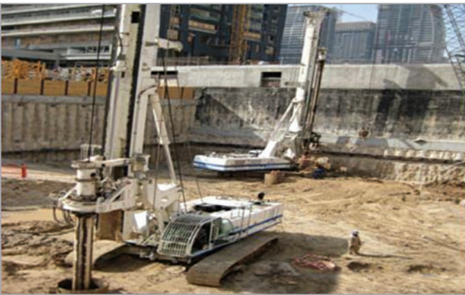
▲ Bored Pile Installation at Dubai.
