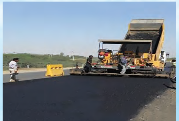
BC laying in progress - Bhuj Bhachau-Kachchh
