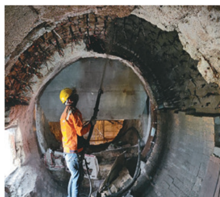
▲ DURAGUN application in progress in cement plant
